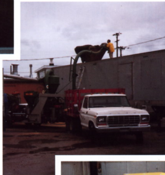
A 45-foot trailer containing the entire bag filling operation being loaded pneumatically
